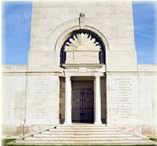
Doors to the Tower at the Australian National War Memorial
