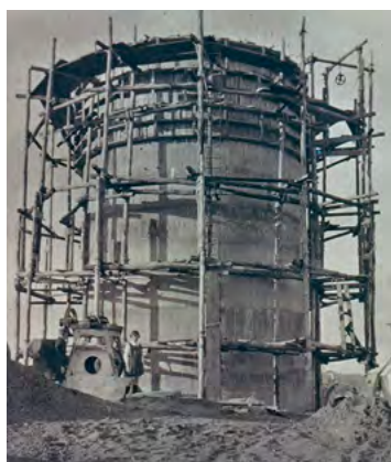
Berwick Water Tower construction 1926
