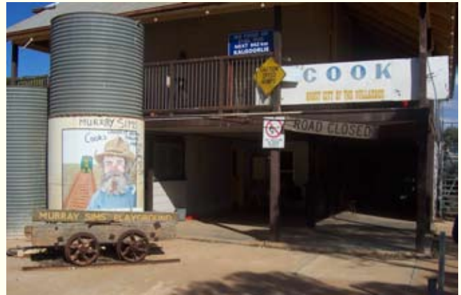
Abandoned building in Cook. Mural to longest serving railway worker 28 years.
